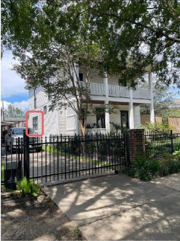
VIEW OF WINDOW FROM TULANE ST
